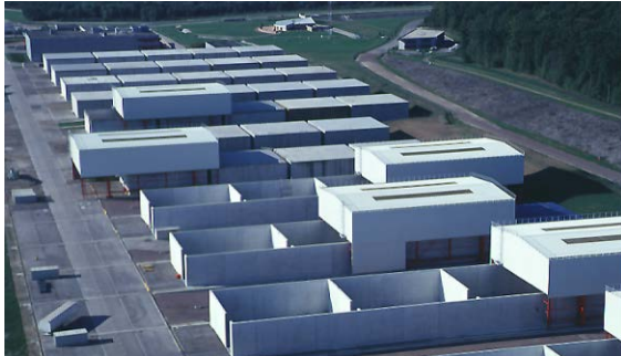
Figure 2: changes in the design of disposal vaults. In the background first generation separate vaults, in the foreground grouped vaults on a single bottom slab
