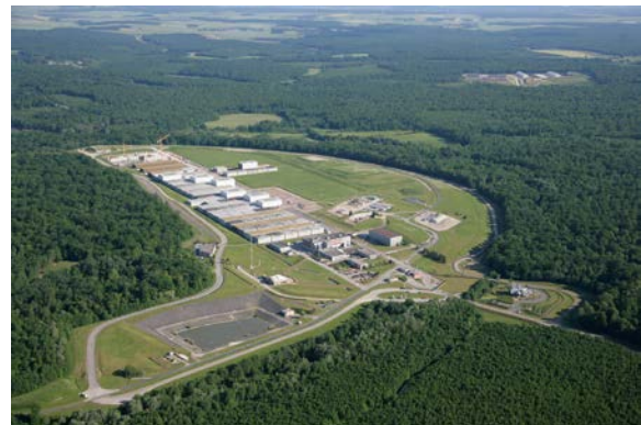
Figure 1: general view of centre de l'Aube disposal facility
