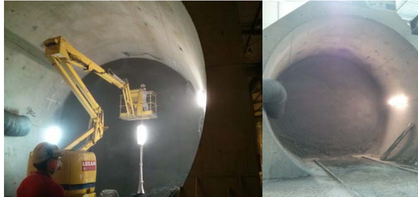
Fig. 10 - The low pH shotcrete containment wall construction (spraying/ left; end product/right)
