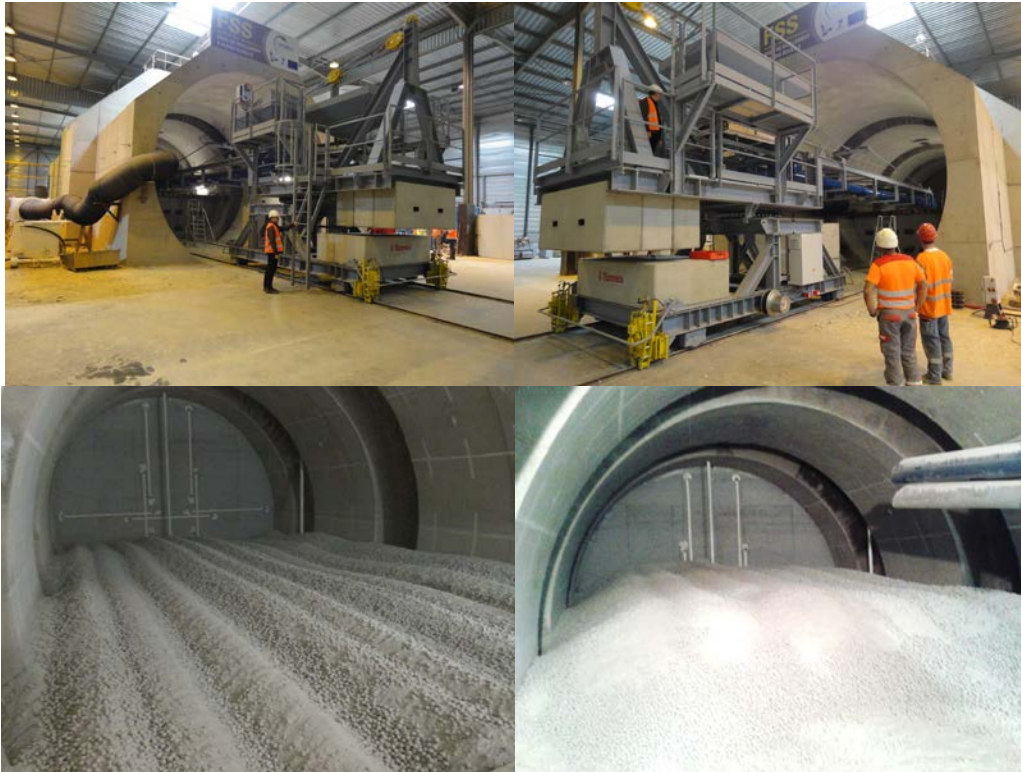
Fig. 9 - The swelling clay core emplacement operations
