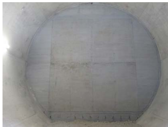
Fig. 7 - The low pH SCC containment wall as an end product
