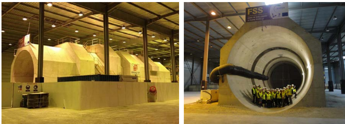
Fig. 4 - The FSS test box ready for seal construction
