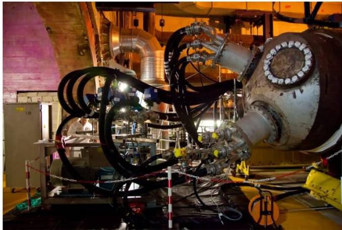
Fig. 4. Connexion of a SG to the AMDA© (Automated Mobile Decontamination Appliance) deployed by AREVA NP to apply the CORD© process.
