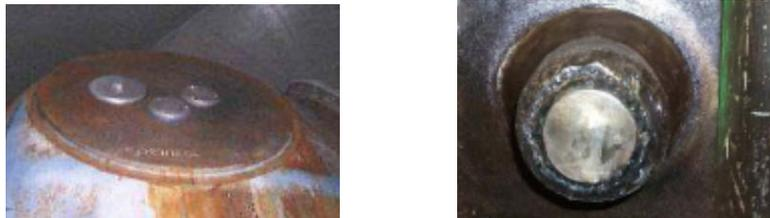
Fig. 6. Illustrations of the sealed orifices: cover plates and plugs.
