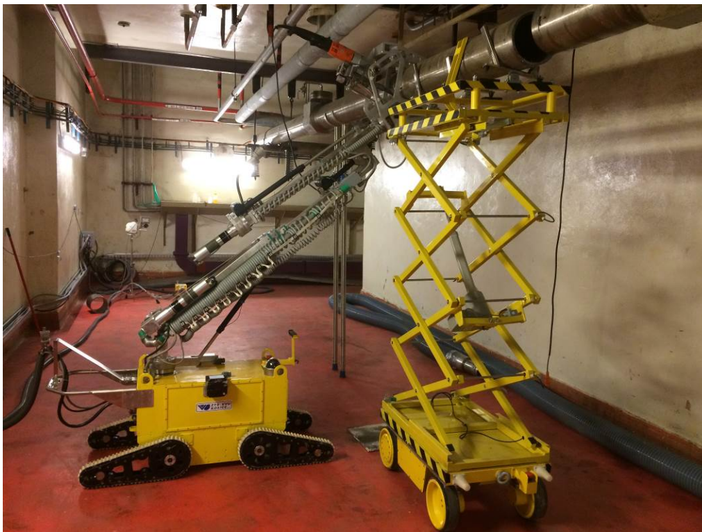
Figure 6. Manipulator MT15 in operation
