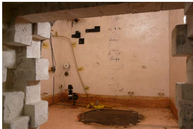
Figure 3. Room 200 after dismantling
