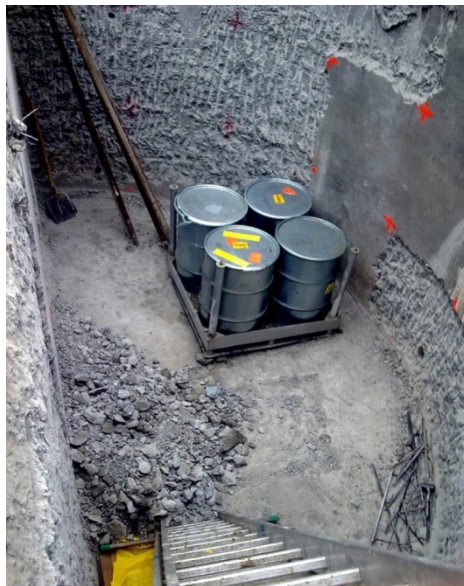
Fig. 3 Hammering of the inner concrete surfaces
