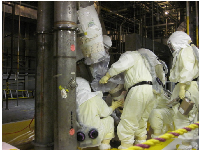
Figure 1: Crews removing ventilation ductwork, heavily contaminated after years of plutonium production.
