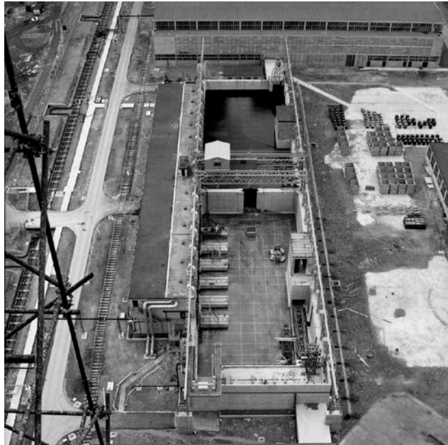
Fig. 1. Pile Fuel Storage Pond during construction
