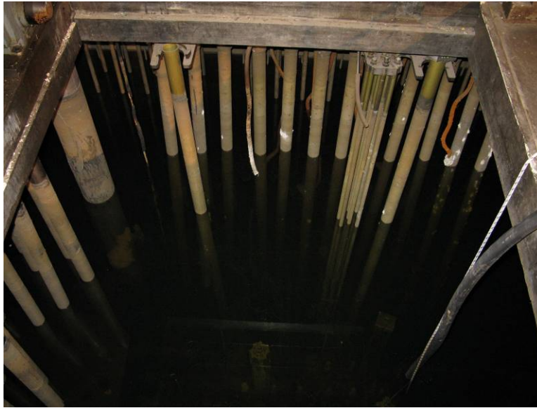
Fig.2 Reactor MR pond after dismantling truck of control and protection system and movable fuel assembly.
