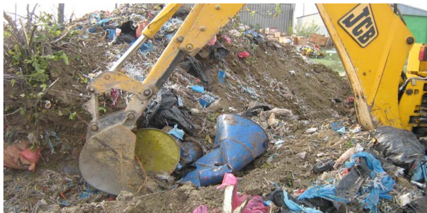
Fig. 3. Inadequately buried radioactive wastes.
