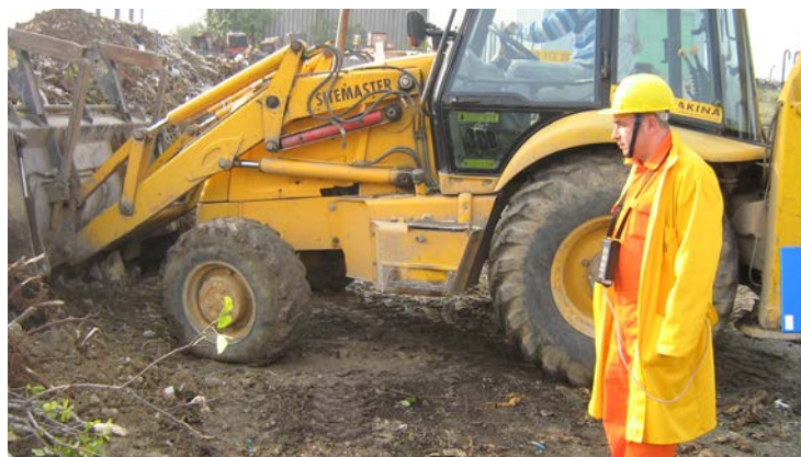
Fig. 2. Removal of radioactive waste from inadequate disposal area.
