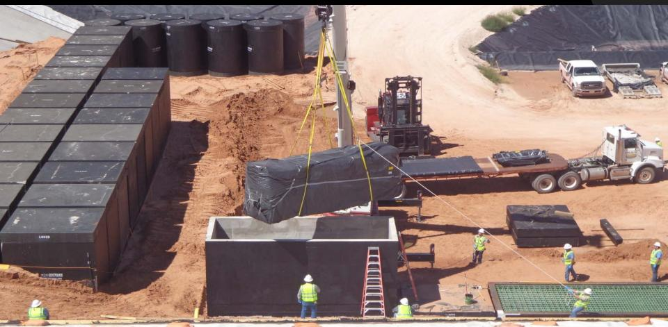
WCS workers place a MLLW Class C oversized component into a custom MCC for final disposal. This disposal method provides the generator and WCS workers with significant ALARA benefits by not having to size reduce the component for final disposal.
