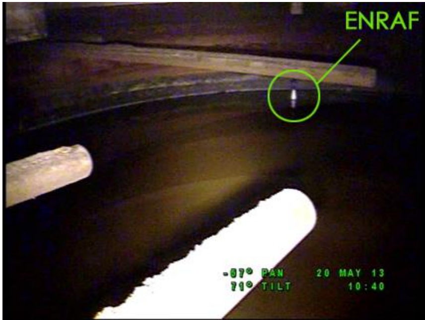
View inside tank T-111 with ENRAF tank level gauge visible
