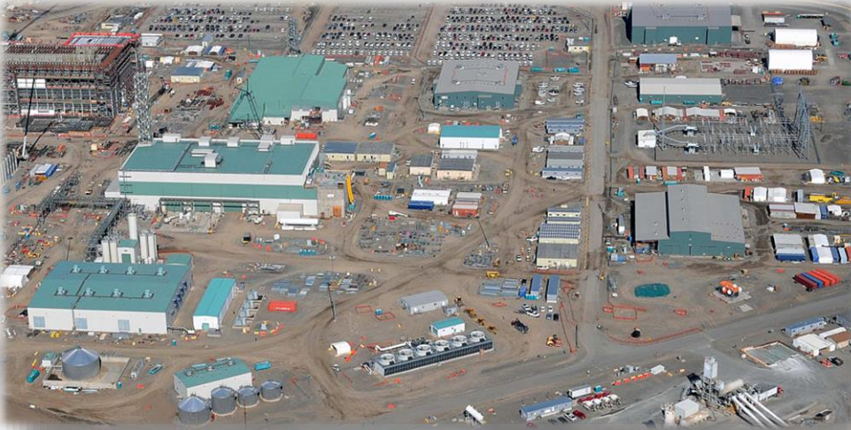
20 support buildings for the Balance of Facilities
