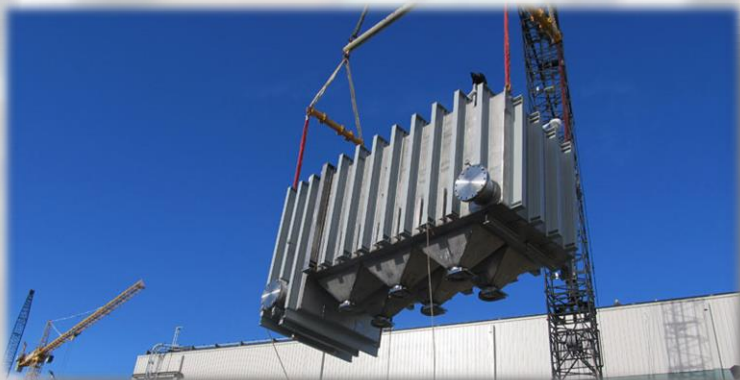
Carbon bed adsorber
