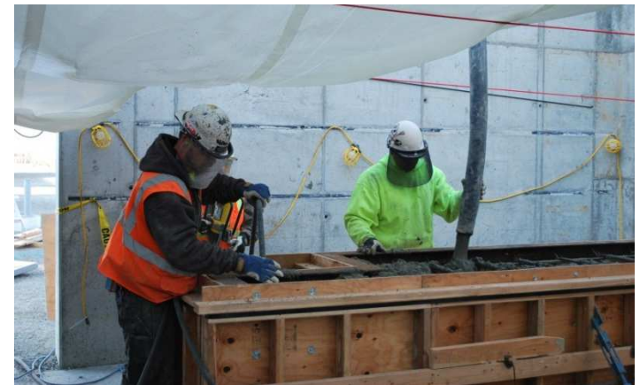
Placing concrete for the KW Annex
