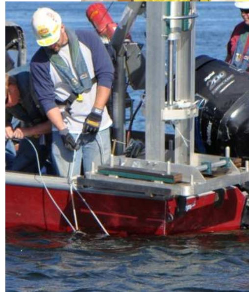
Installing aquifer tubes along the Columbia River
