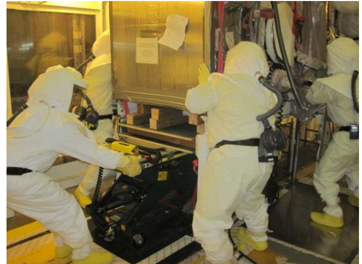
Removing a glovebox from PFP
