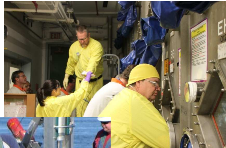
Preparing large pieces of contaminated equipment, called gloveboxes, for disposition at PFP
