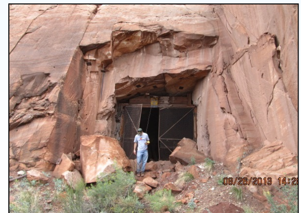
Unsecured mine opening
