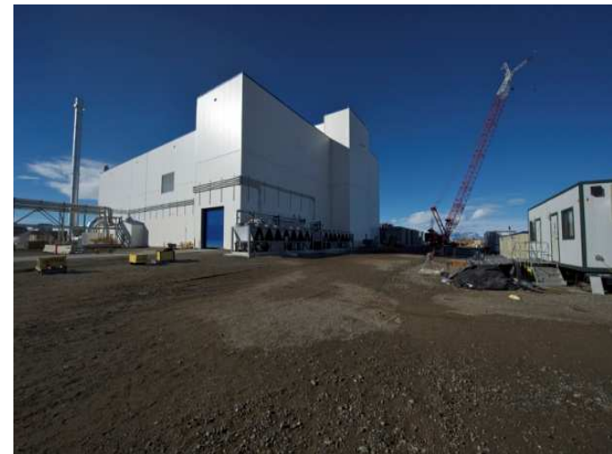
Sodium Bearing Waste Facility
