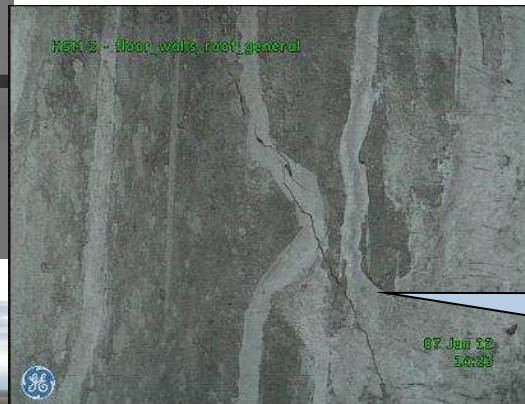
Crack in Horizontal Storage Module wall
