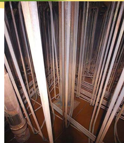
Savannah River Tank 5 Heel Removal (Tank Interior)
