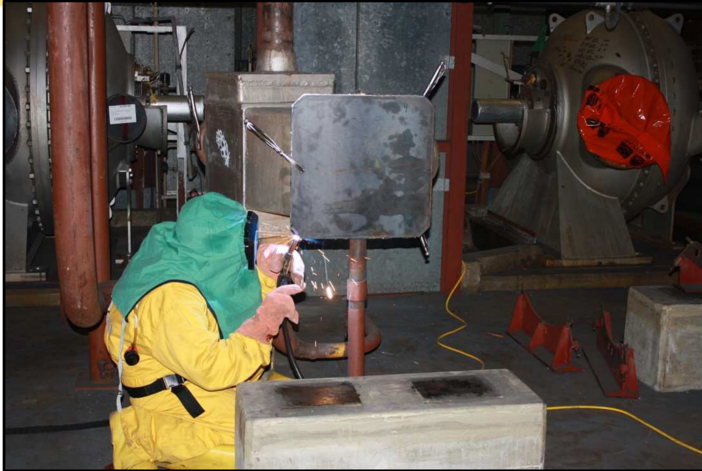
Process gas cooler being removed from the Freon and process gas systems
