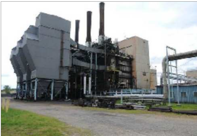
Steam Plant Before
