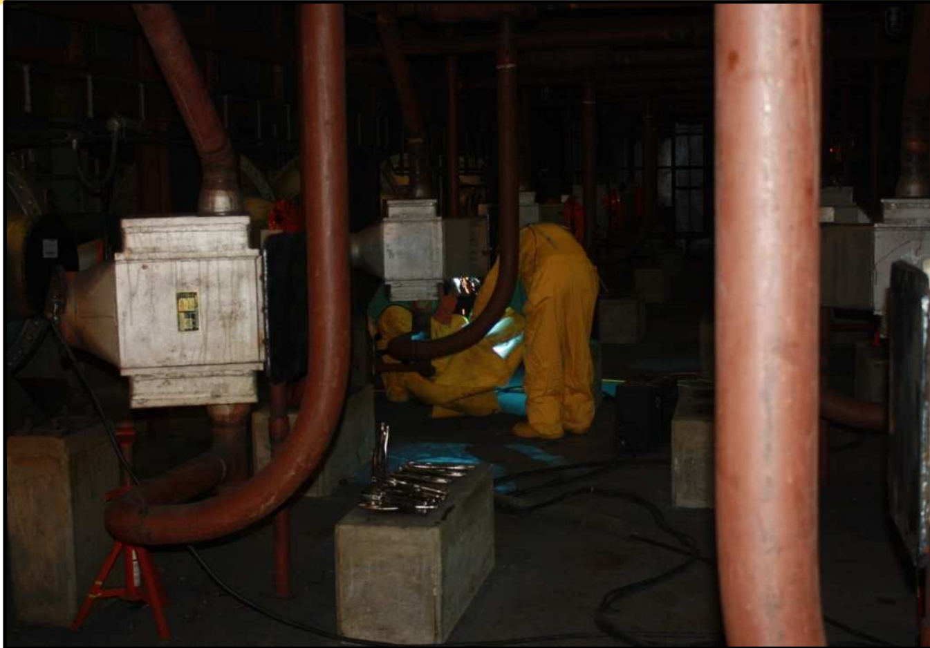
Process gas cooler being removed from the Freon and process gas systems
