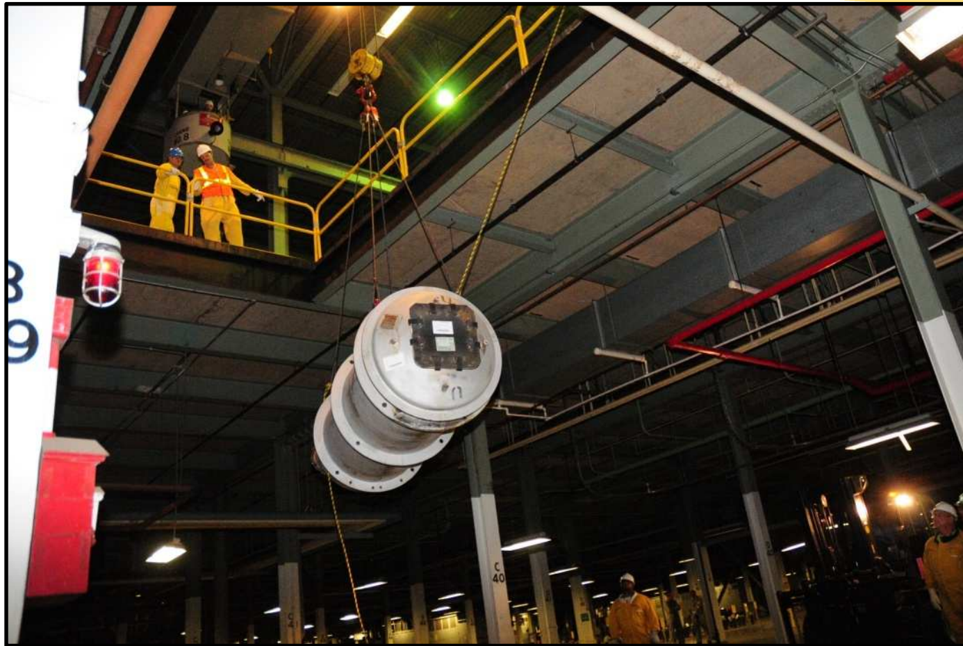
Converter is lowered to the operating floor
