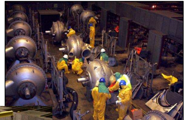
Cut & Cap Operations in X-326 Building
