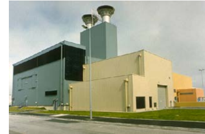
AREVA - La Hague facilities
