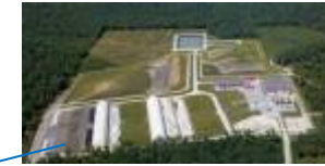
Centre de stockage TFA (CIRES Morvilliers)
