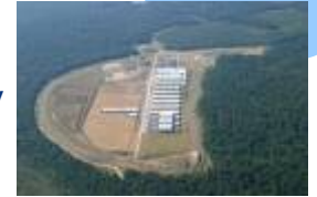
Low and intermediate level Waste repository (CSA Soulaire)
