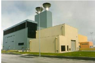
Areva - La Hague facilities
