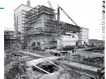
Magnox repro' under construction
