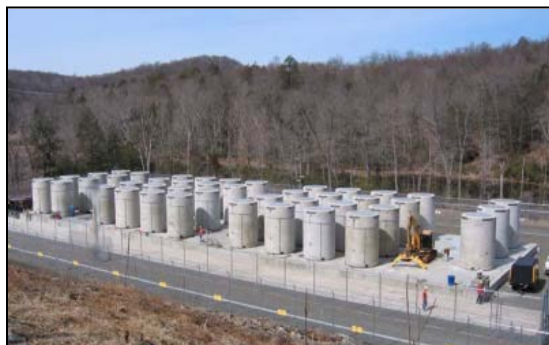
Typical Cask Storage Facility
