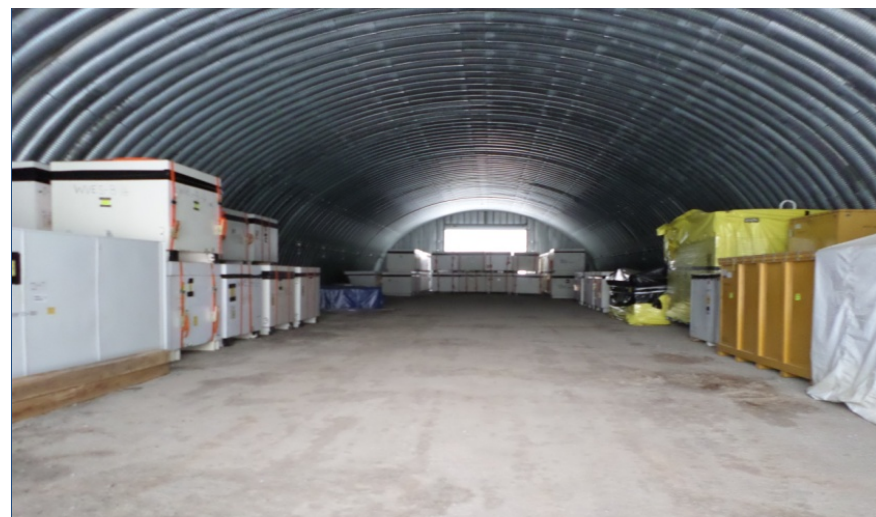
Packaged TRU Drums in CPCWSA Storage
