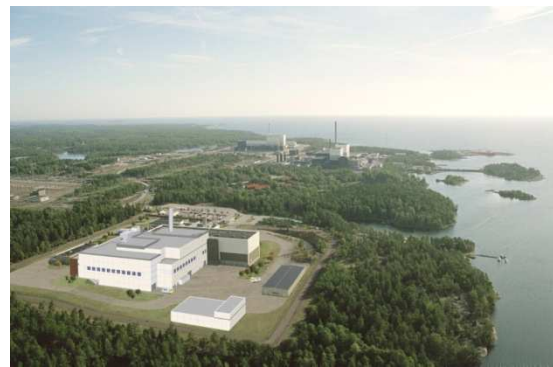
Encapsulation plant in Oskarshamn
