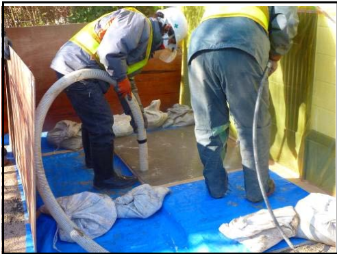
High pressure water cleaning of paved road
