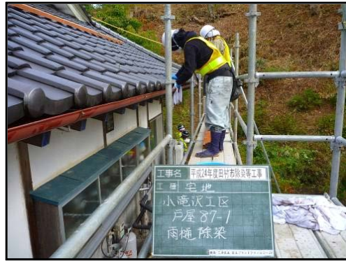
Wiping off a gutter
