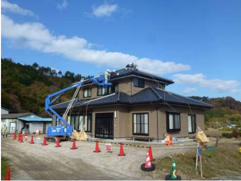
Wiping off rooftop and walls
