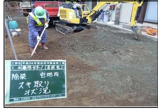
Removal of crushed stones and topsoil, and cover with clean soil
