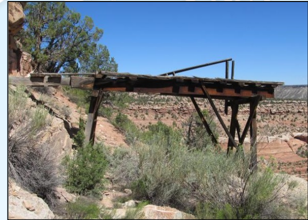
A timbered load-out trestle associated with a small adit in the Uravan mining area of Colorado.
