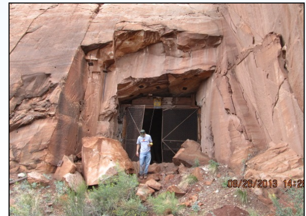
Unsecured mine opening
