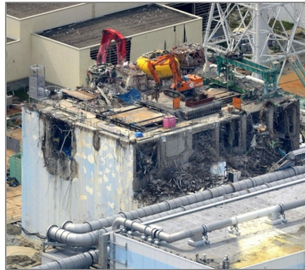
Debris Removal from Unit 4
