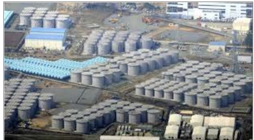
Fukushima Daiichi NPS Tank Farms
