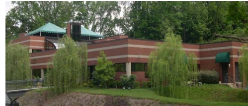
Perma-Fix Business Center Knoxville, TN
