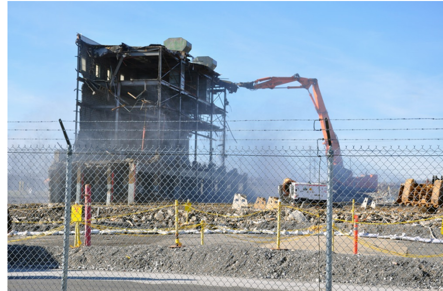
K-25 Demolition Completion
