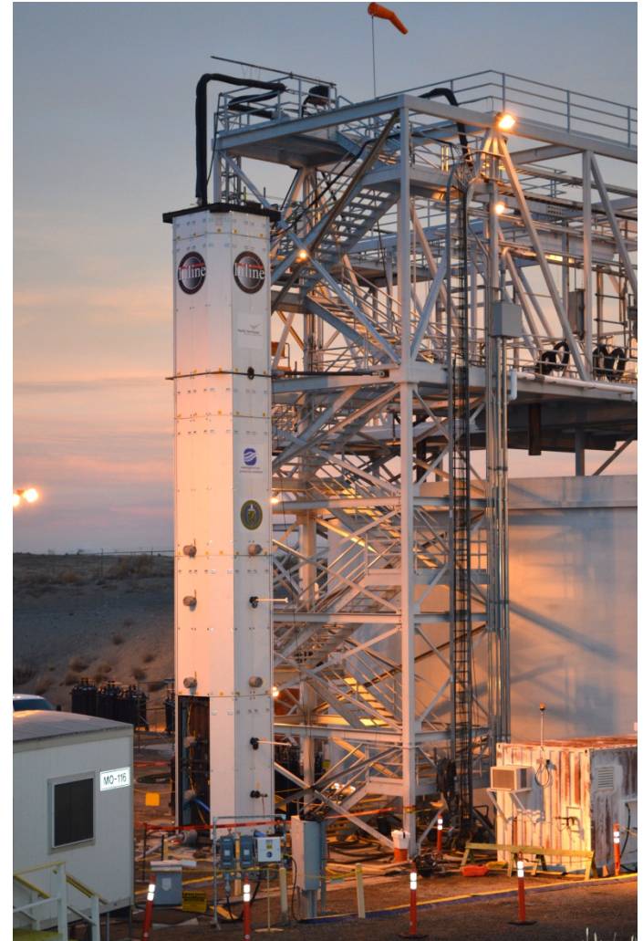
Potential gas release event testing
