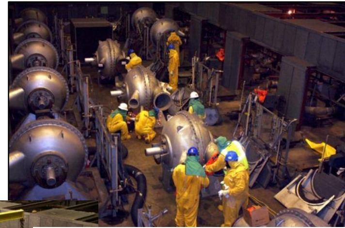
Cut & Cap Operations in X-326 Building
