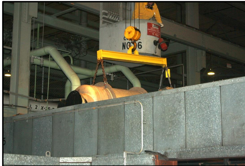
Converter is raised from the cell using the crane
