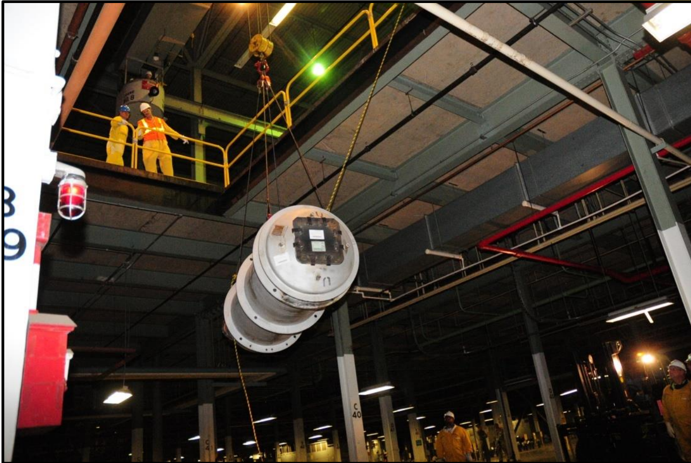
Converter is lowered to the operating floor
