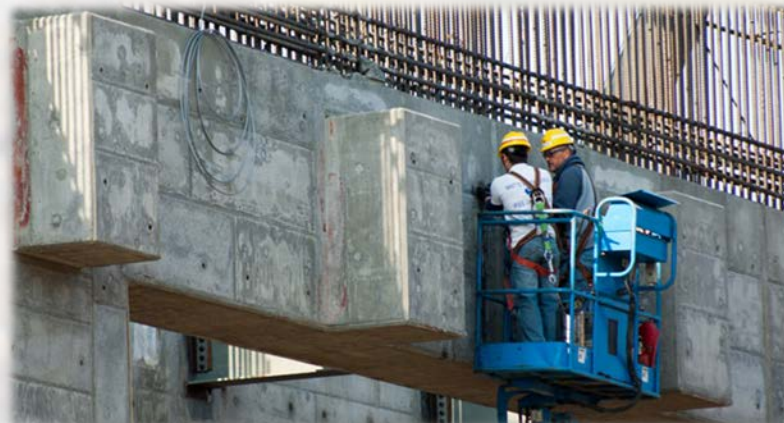
Truck Bay Walls
