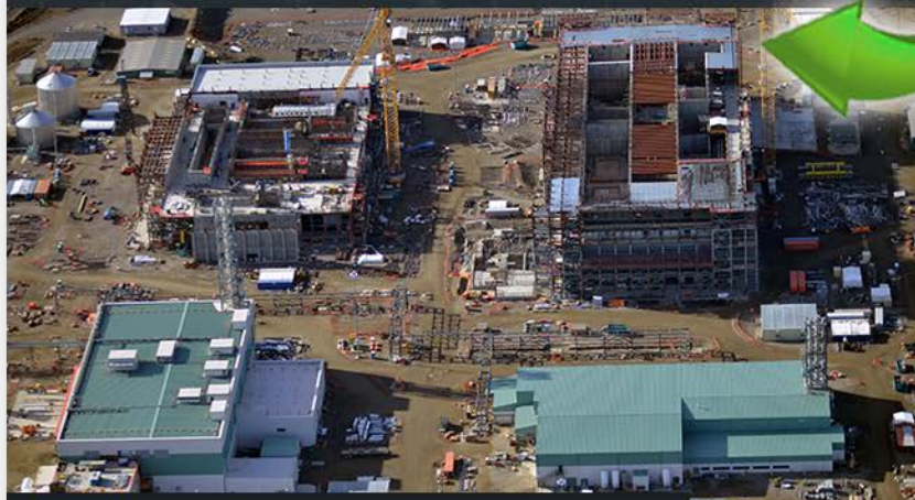
Present: Waste Treatment Plant Construction
