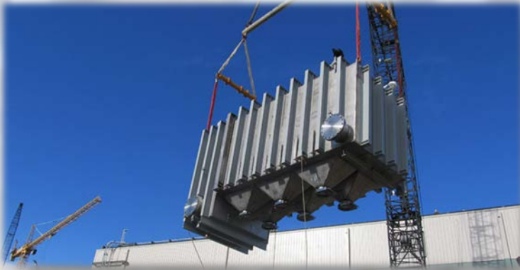
Carbon bed adsorber
