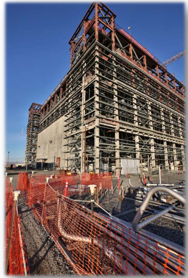
Structural steel frames a corner of the Pretreatment Facility
