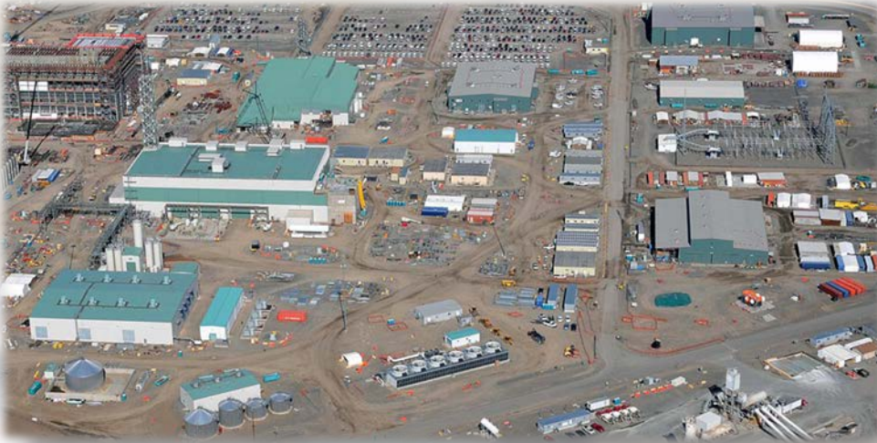
20 support buildings for the Balance of Facilities
