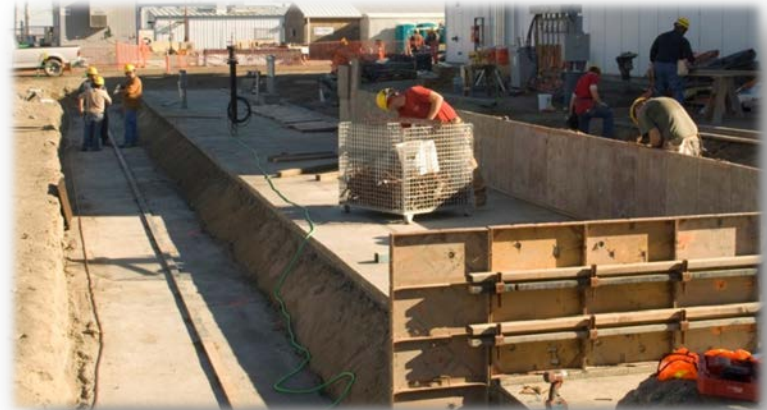
Balance of Facilities employees continue building the foundation for the emergency power generators
