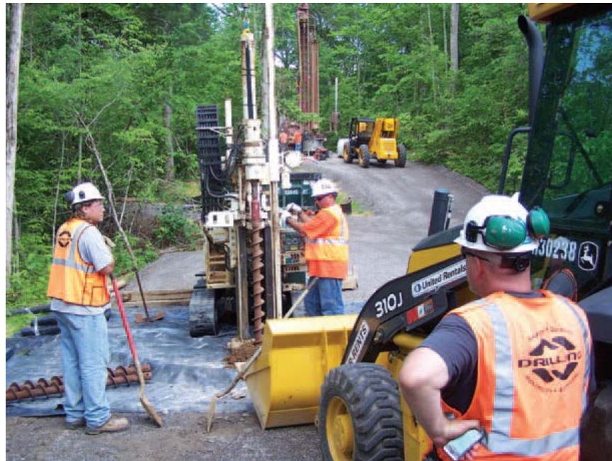
Installing monitoring wells along Raccoon Creek
