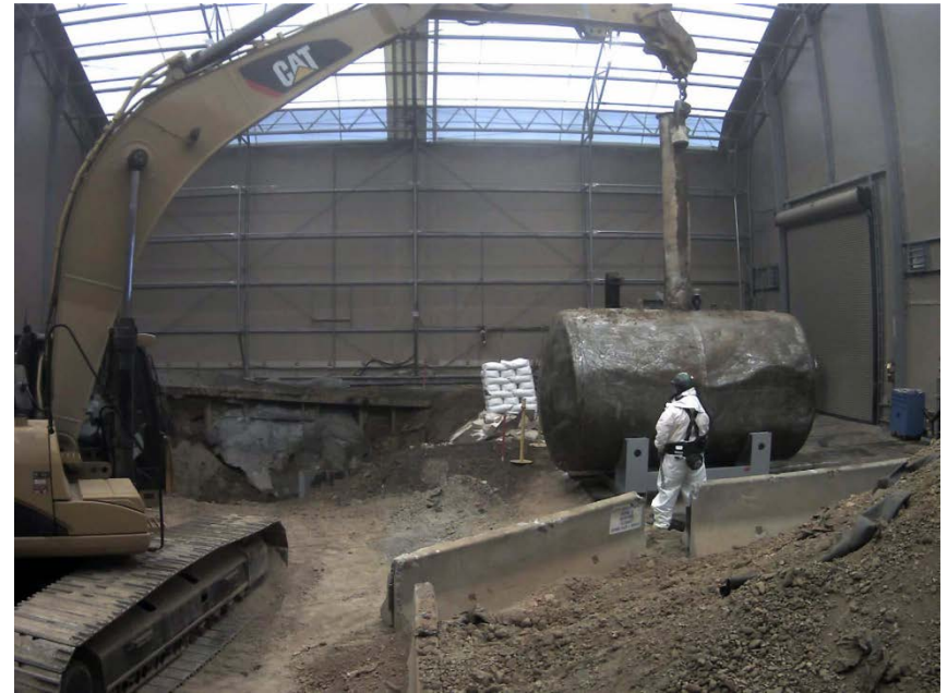
Tank W-1A in Bethel Valley being removed from the ground
