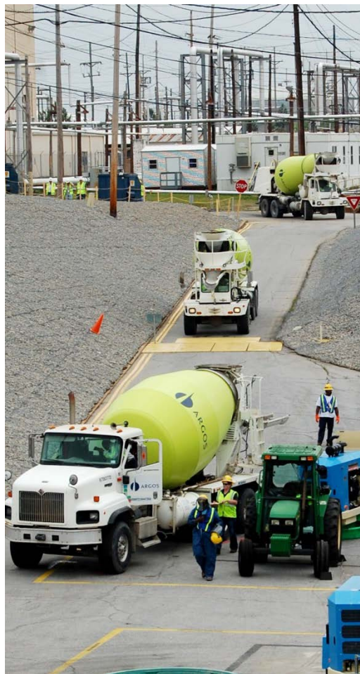
Pouring grout into SRS waste tanks (April 2012)
