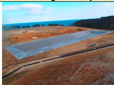
Bottom of soil covered temp, facility
