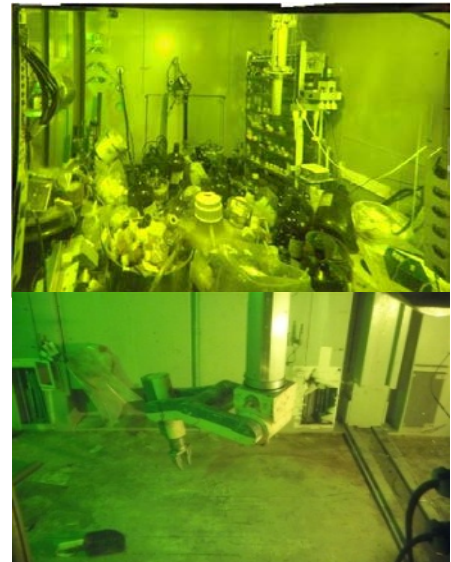
Building 205 K-Wing Hot Cell (A-Cell) in 2009 (Top) and 2011 (Bottom).
