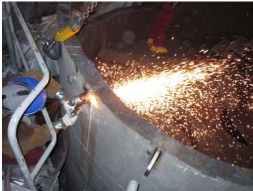
Fig. 11. Steam Generator Segmentation.
