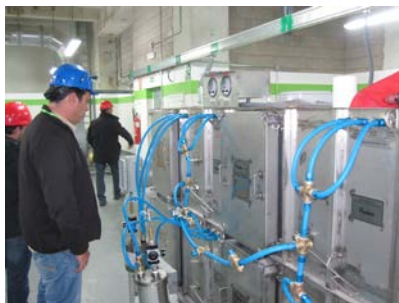
Fig. 15. EAD Ventilation Equipment (Testing).
