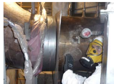
Fig. 20. Primary Circuit Isolation.
