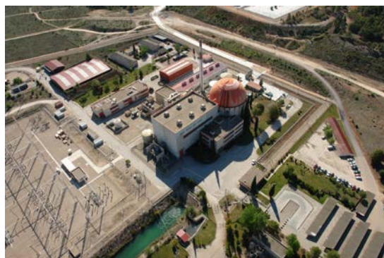
Fig. 2. José Cabrera NPP General View.
