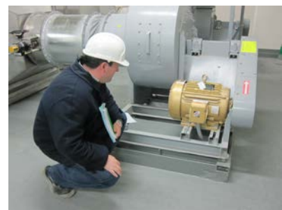
Fig. 16. EAD Ventilation Equipment (Testing).
