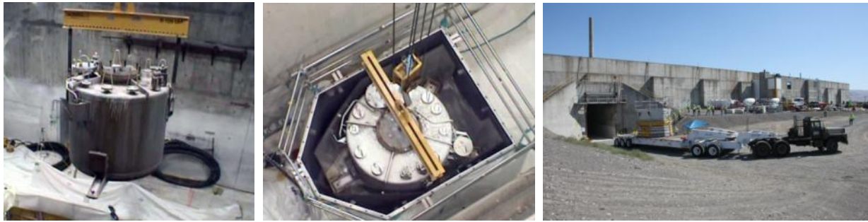
Figure 1 Removal of Tank D-10 from U Canyon
