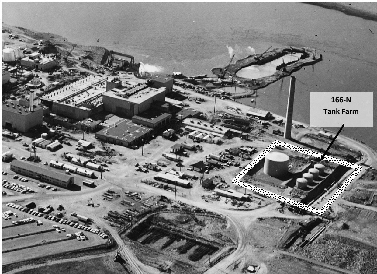
Fig. 1. 166-N Tank Farm Facility (Early 1960s).
