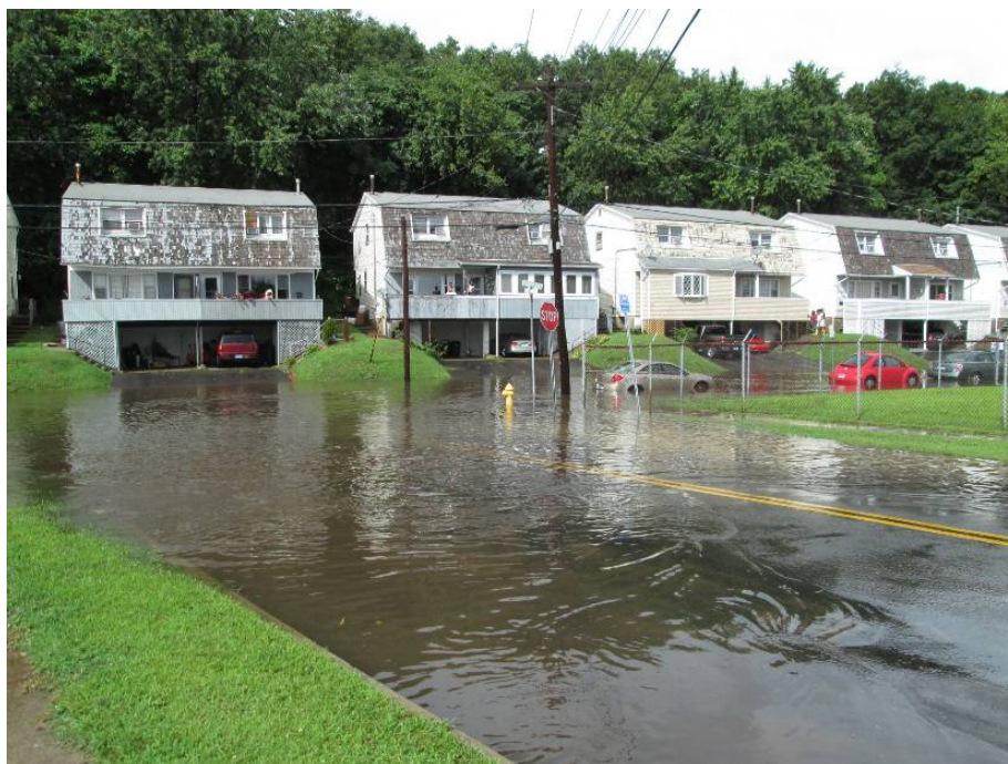
Figure 7: Street flooding in a portion of the neighborhood with inadequate storm drainage.
