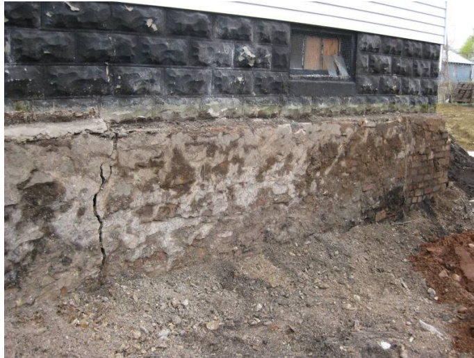
Figure 6: Photo showing crack in foundation constructed of stacked stone and brick.
