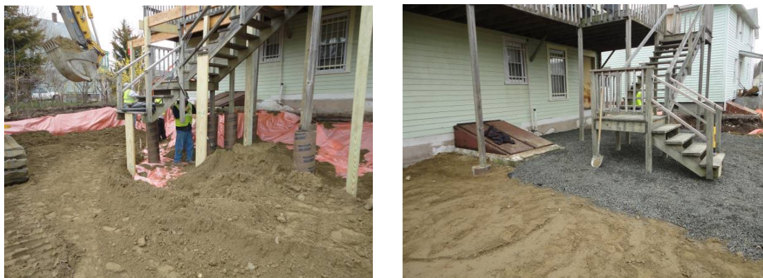
Figure 4 and 5: Excavation and backfill around a three story staircase. This work was completed in one day to allow safe access to apartment on the 2 nd and 3 rd floors.
