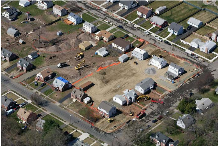
Figure 3: Aerial view of one block during excavation and backfill
