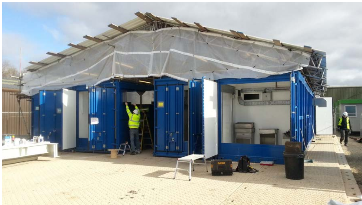
Modular Liquid Effluent Treatment Plant during final assembly
