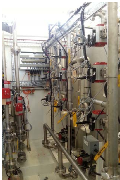
Ion Exchange Skid
