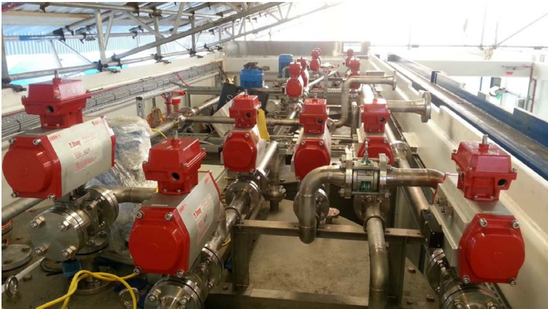
Top Mounted Motorised Valves for ease of maintenance
