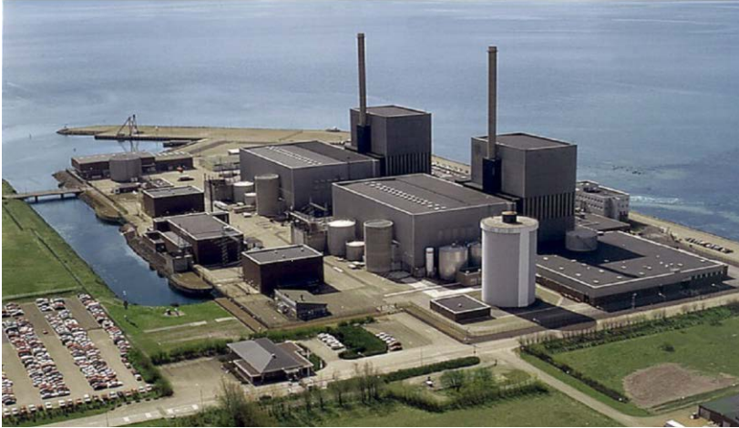
Picture 1 Barsebäck NPP in Sweden
