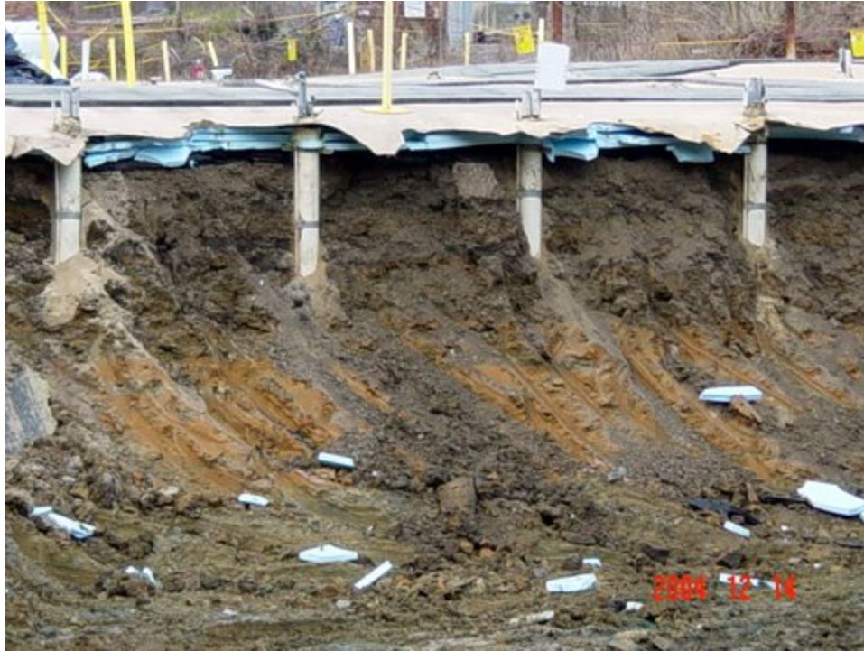
Fig. 6: Exposed Frozen Soil Thawing in December 2004
