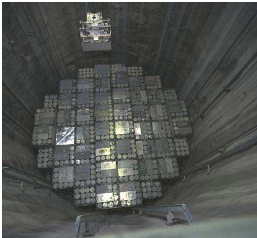
Fig. 3. View to the low- and intermediate level waste silo at the Olkiluoto repository (Source: TVO).
