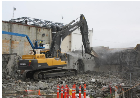
Demolition of the Turbine Building First of Five Major Civil Works Projects Underway
