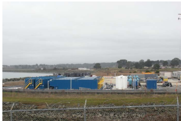
Installation of the new GWTS completed 2013
