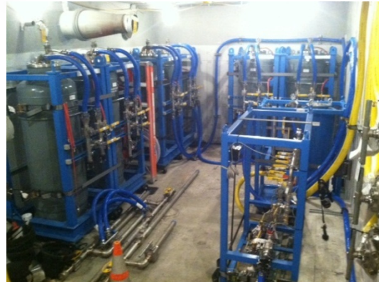
FIXS installed inside Refueling Building
