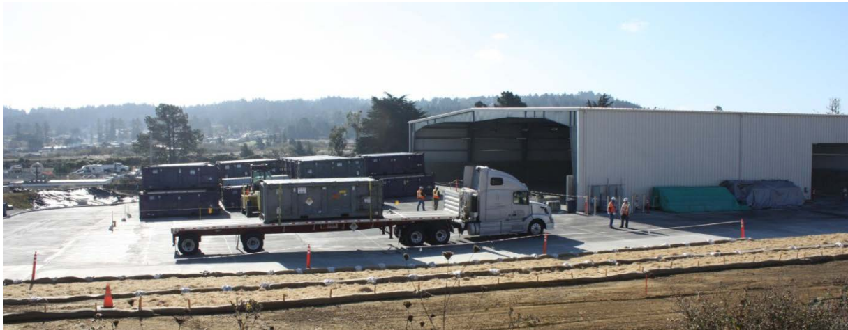
Newly Constructed Waste Management Facility where Fossil Units Bulk Storage Tank Resided
