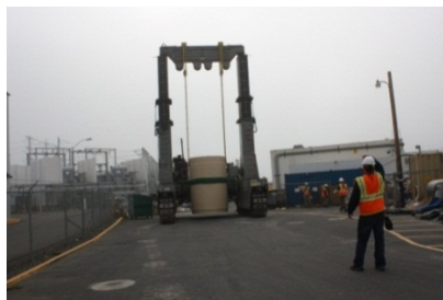
VCT Transporting GTCC Cask 6
