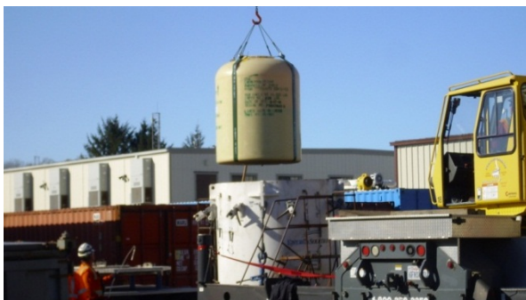
B/C Waste being loaded in Energy Solutions Cask
