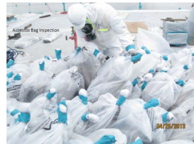
Turbine Building asbestos abatement generated more than 350 bags
