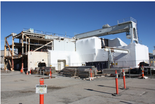
Demolition of the Turbine Building First of Five Major Civil Works Projects Underway
