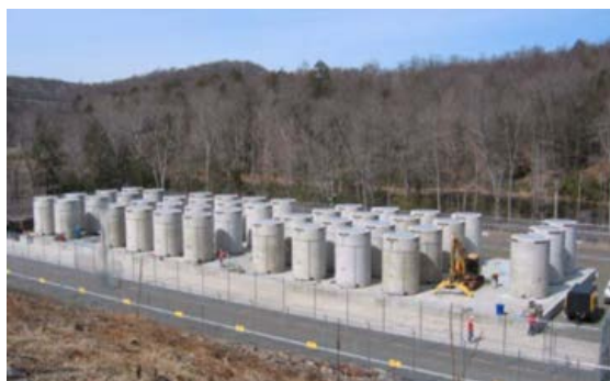
Picture 3 A typical ISFSI for spent fuel dry storage.
