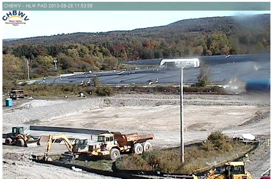
Picture 4 Completed excavation of the storage pad (up to 15' deep)
