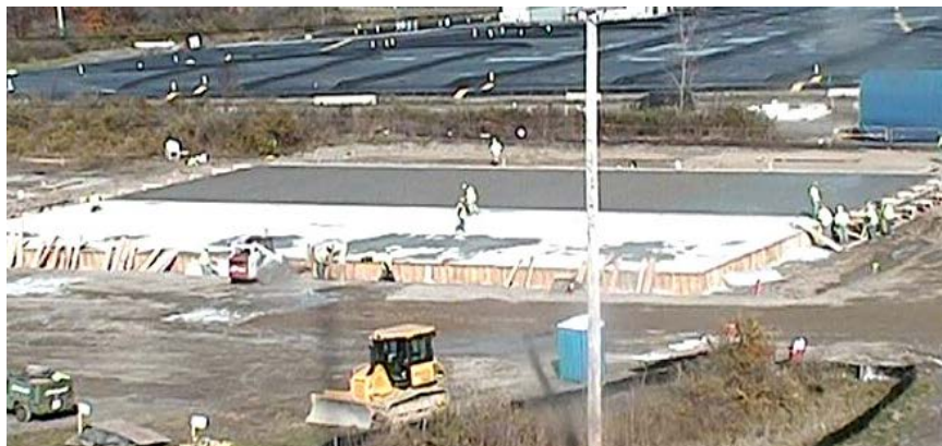
Picture 7 The constructed storage pad.
