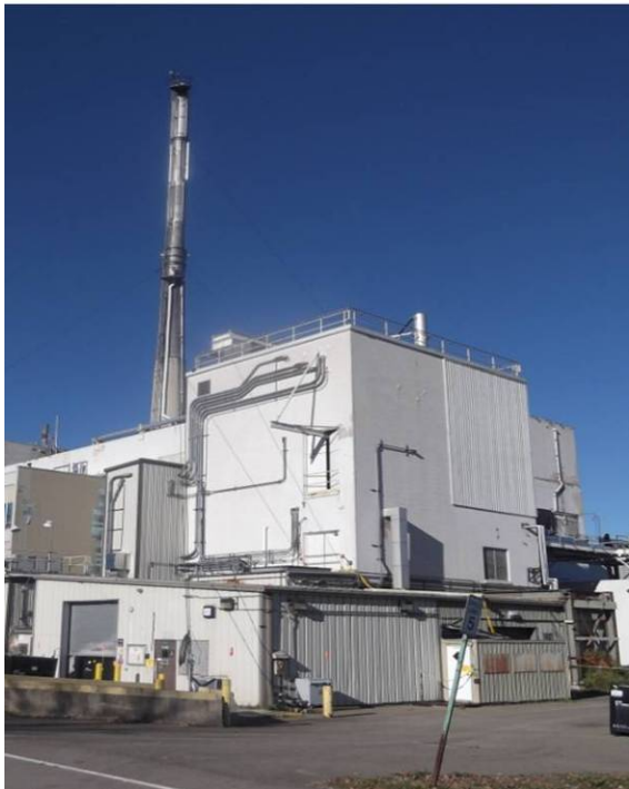
Photo 1 - The 01-14 Building, prior to the start of demolition
