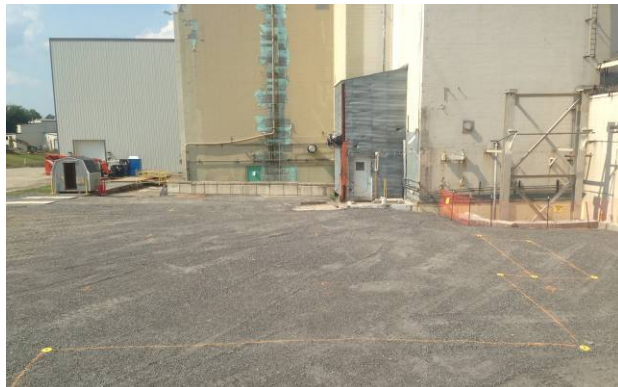
Photo 5 – The 01-14 Building slab covered with backfill.
