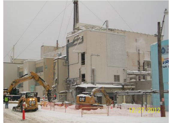
Photo 2 – Phase 1 demolition of the 01-14 Building.
