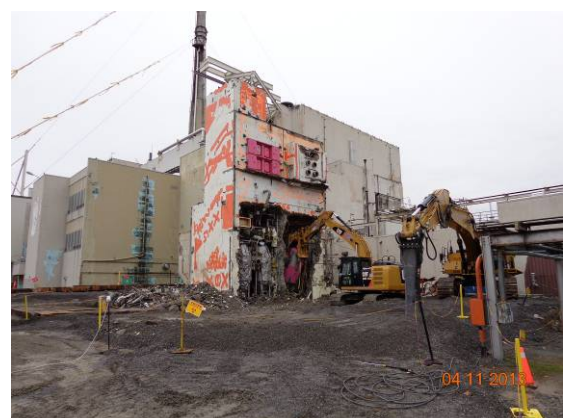
Photo 4 – Phase 3 demolition of the 01-14 Building.
