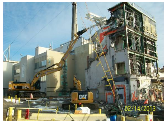
Photo 3 – Phase 2 demolition of the 01-14 Building.
