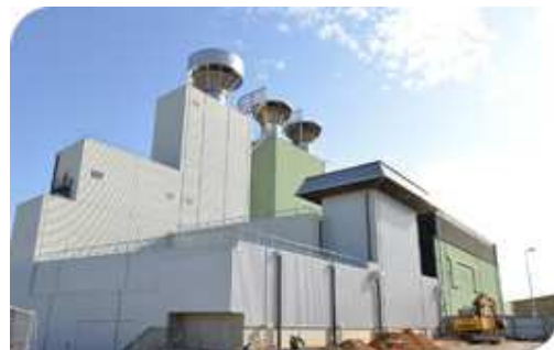
Figure 7 EEVLH facility for HLW storage
