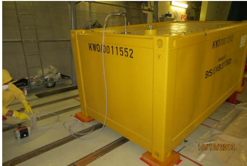
Fig.11 Pumping of free-moving liquids out of the Konrad-Container
