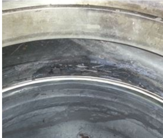
Fig. 9, seating area after securing all cooling and installation of a metallic seal
