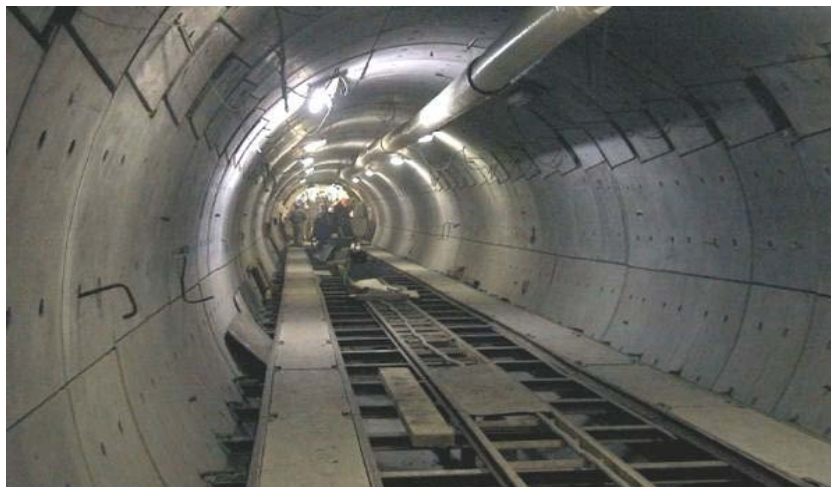
Fig. 2: Connecting gallery of the HADES URF with concrete wedge block lining
