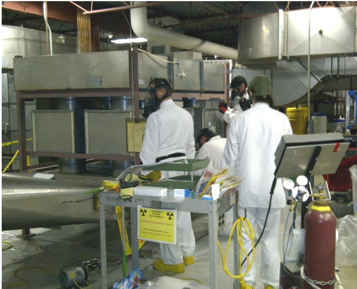
Figure 5. Mixed Trades and RP Preparing to Disassemble HEPA Filter Bank
