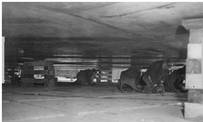
Figure 6 – Workers creating ventilation slots in the Kaolite pedestal once the primary tank has been lifted with cribbing
