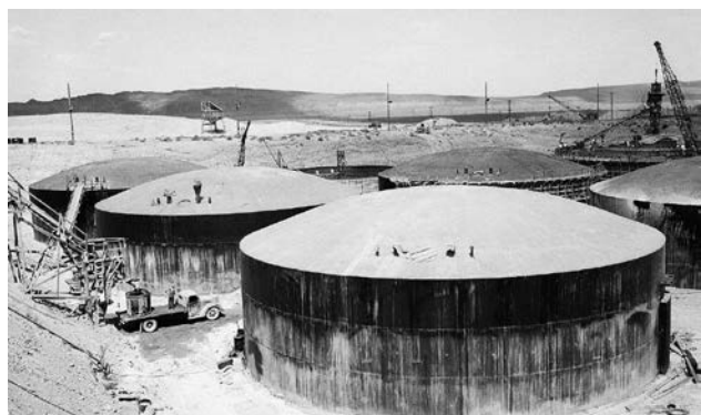
Figure 2 – Construction of the BY Farm SSTs in 1949 2
