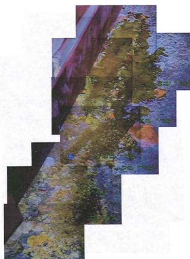
Figure 11 – 241-AY-102 Waste in the Annulus near Riser 83 (November 2012)
