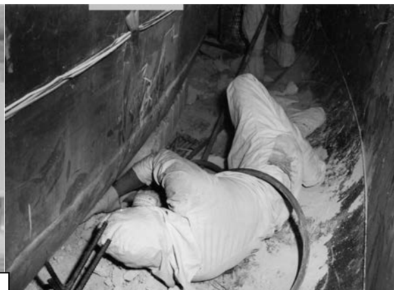
Figure 7 – Workers in the annular space removing 21 inches of Kaolite material under
