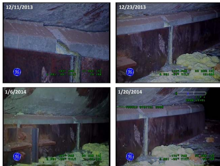
Figure 13 – 241-AY-102 Waste in the Annulus near Riser 83 (Jan 2014)
