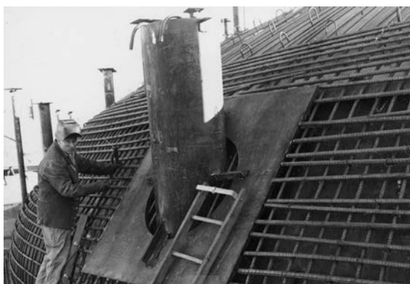
Figure 5 – Worker welding flashing to the risers and surrounding rebar in the haunch region
